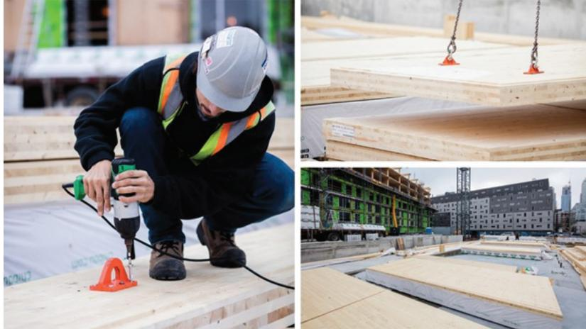
Construction of ARBORA complex with 435 residential units using massive timber in Montreal, Canada. Foto credit: Nordic Structures.
