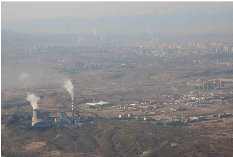
The coal-fired Urumqi Thermal Power Plant in western China.
