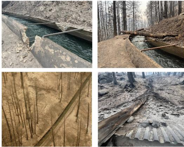
Figure 4: Damage to the Yakima-Tieton Main Canal | Source: Yakima-Tieton Irrigation District
