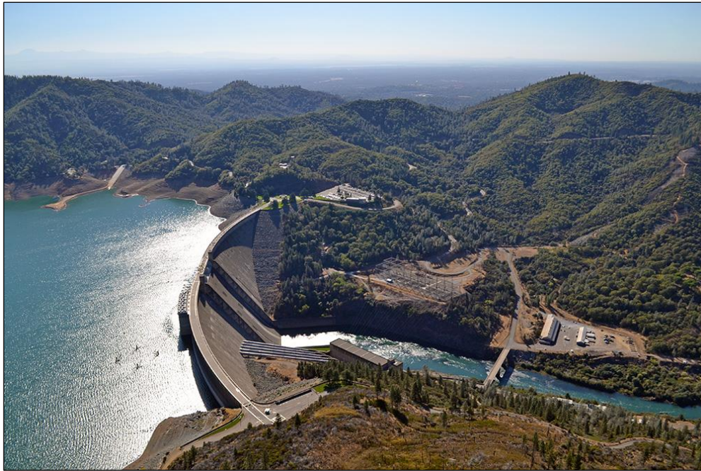
Figure 2. Shasta Dam and Reservoir
