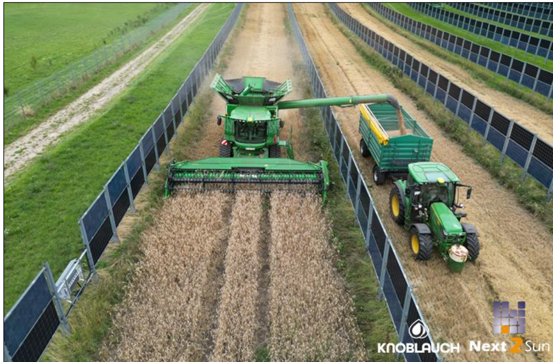
Figure 7. Vertical, Dual-Faced Solar PV Configuration
